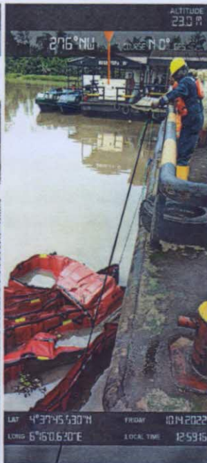
BOOM (ARRANGING & DROPPING OF BOOM ON THE IMPACTED AREA)
